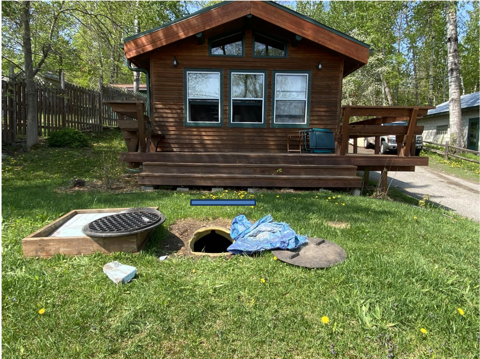
Site photo showing approx. 2 ft requested setback to structure (attached deck)
