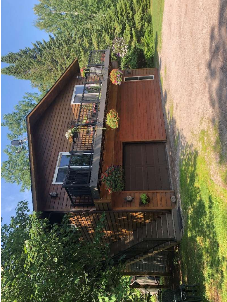
Existing Dwelling – driveway side
